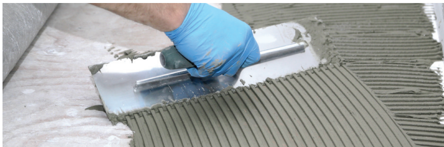
FIGURE 2.12: Spread thinset onto subfloor
