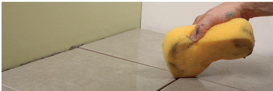
FIGURE 2.23: Clean grout lines
