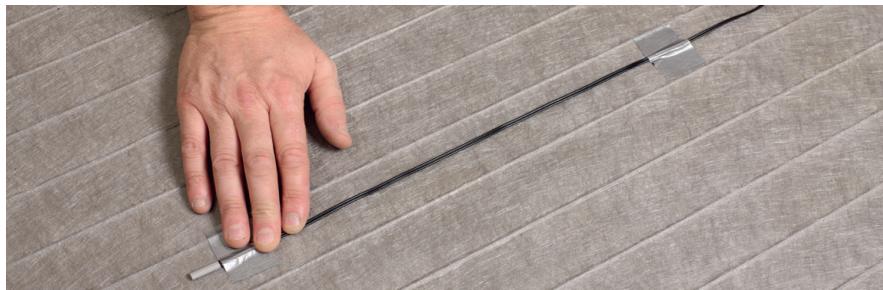
FIGURE 2.16: Secure floor sensor probe
