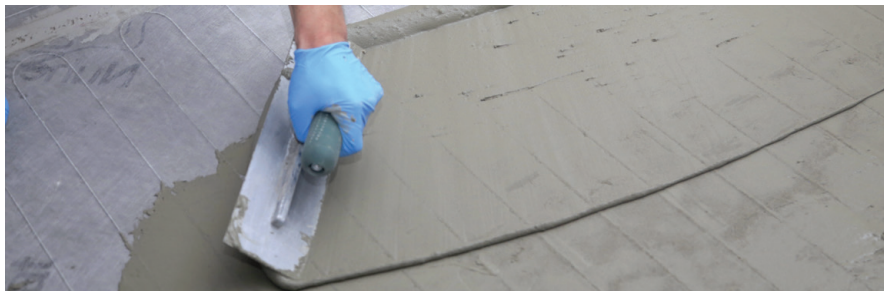
FIGURE 2.21: Install tile/stone flooring
